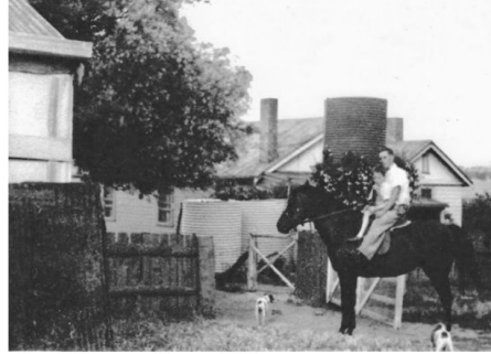
Rear of Charnwood house, 1954
