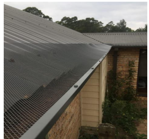
Bushfire mesh on a gable roof (Infodec Communications, 2019).
